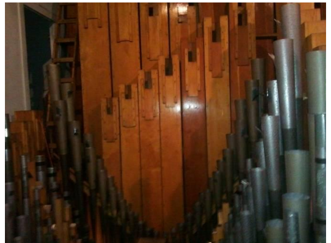
Pipes that have already been clean and tuned and installed back in the pipe loft
